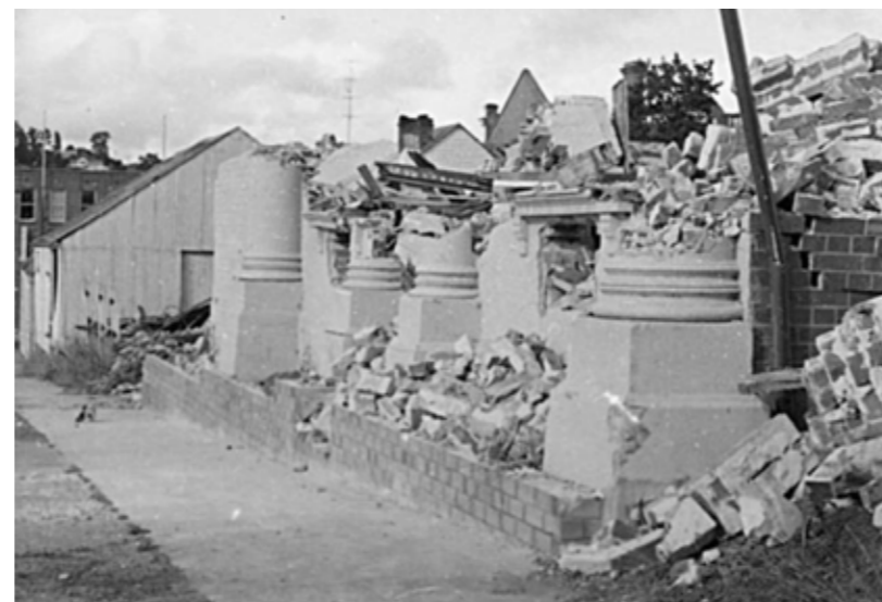
1967 demolition of Olympic Hall, Jessie Street for Woolworths carpark.
