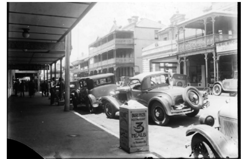
Beardy Street showing wide, weather protected footpaths and in-tact heritage facades.
